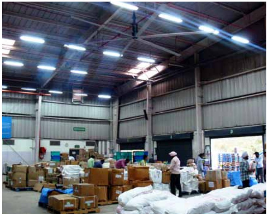
One of Kelley’s “High Volume Low Speed Fan” working in a large warehouse in Punjab.
